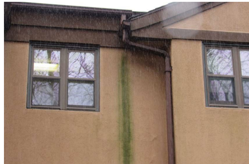
View of discoloration/moisture staining on EIFS cladding as seen at rear of building – appears to be due to failed downspout/gutter
