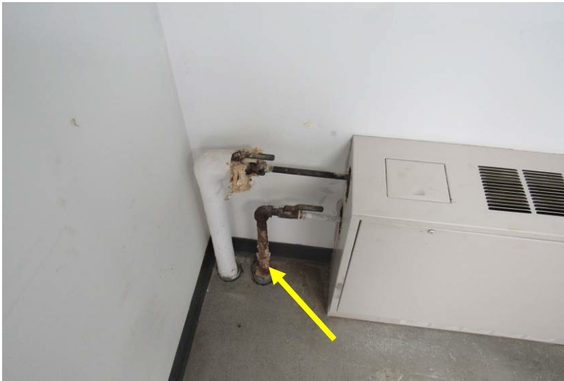
View of pronounced corrosion of hydronic heat copper distribution piping as seen at stairway cabinet heater – sections of distribution piping have been replaced in the past due to failure (common areas and apartment units)
