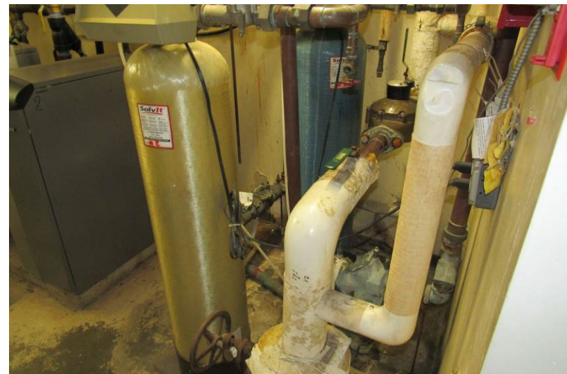
View of water softening system serving development – currently offline for several years
