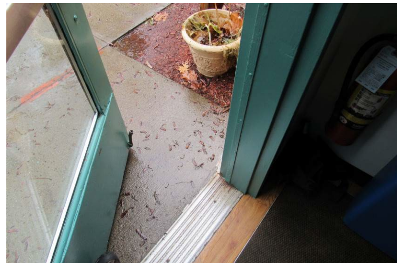
Majority of exterior doorways exhibit corrosion at door frames, abrasions, and finish wear
