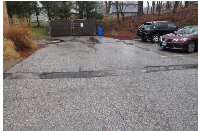
Additional view of pattern cracking/deterioration within asphalt pavement
