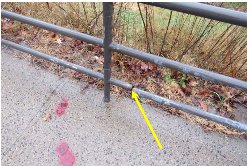
View of section of metal railing at walkway leading to bus shelter/Simeon Road exhibiting damage/wear
