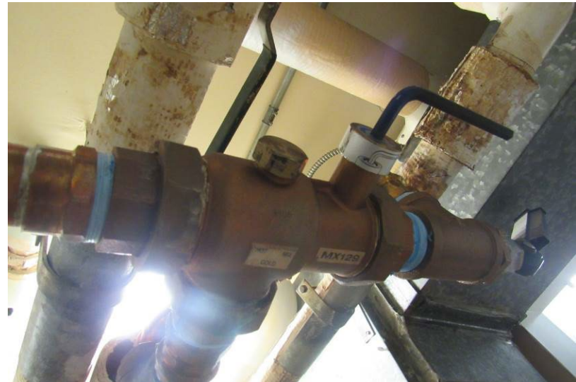
View of domestic hot water mixing valve assembly
