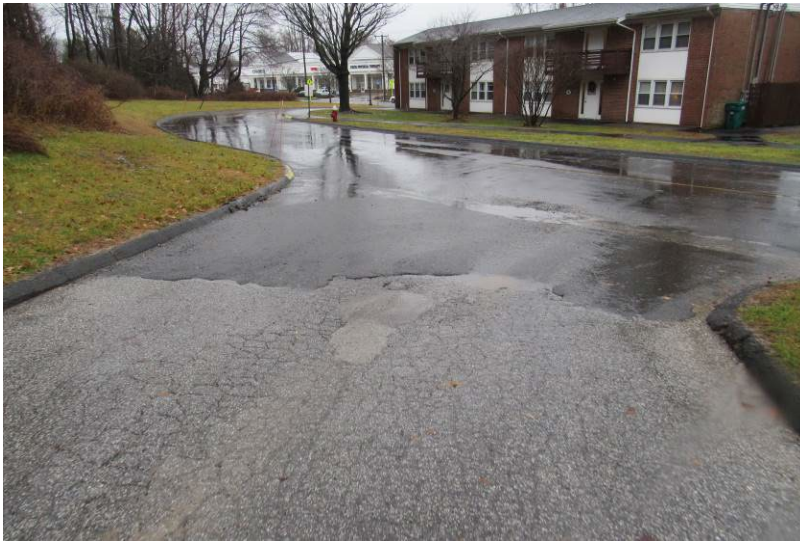
View of pattern cracking and evidence of fatigue within asphalt pavement as seen at entry roadway
