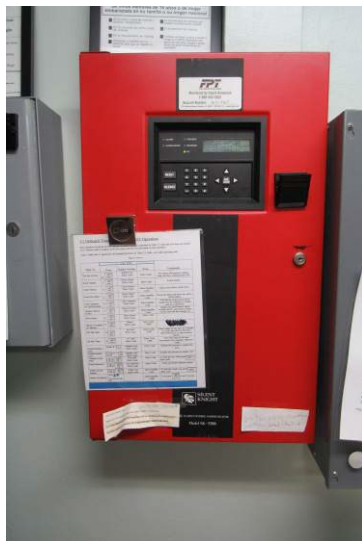
View of Silent Knight SK-5208 fire alarm control panel monitoring hardwired end devices at building
