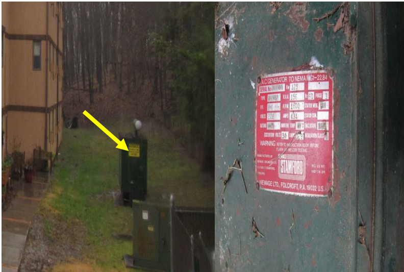
View of diesel-fueled emergency generator present at rear of building and serving key building systems in the event of a power failure – 125 kW rating – diesel fuel is stored in a 2,000-gallon underground storage tank
