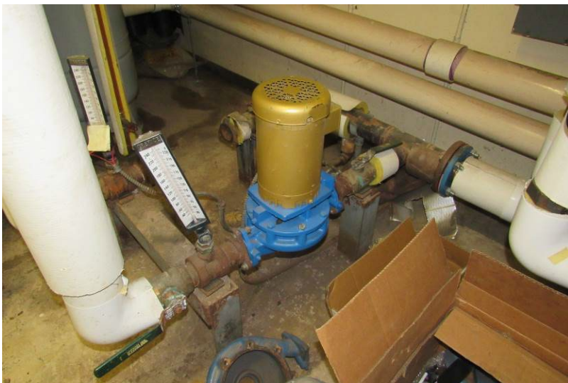
View of vertically-mounted hydronic heat circulation pump, 2-horsepower rating, 86.5% efficiency – motor replaced in 2021 and pump reportedly rebuilt; second pump requires replacement (difficultly obtaining quotes reportedly by management)
