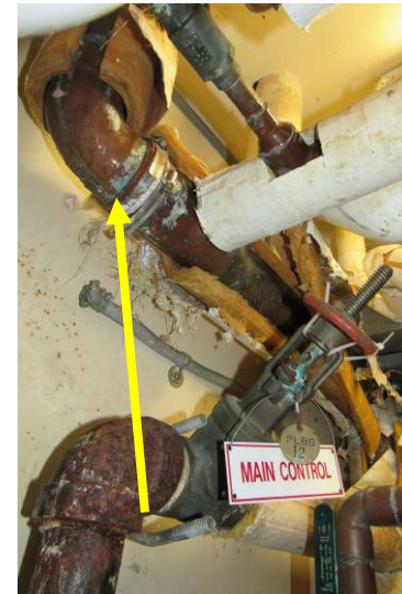
Active domestic water supply piping leakage issues occurring within boiler room
