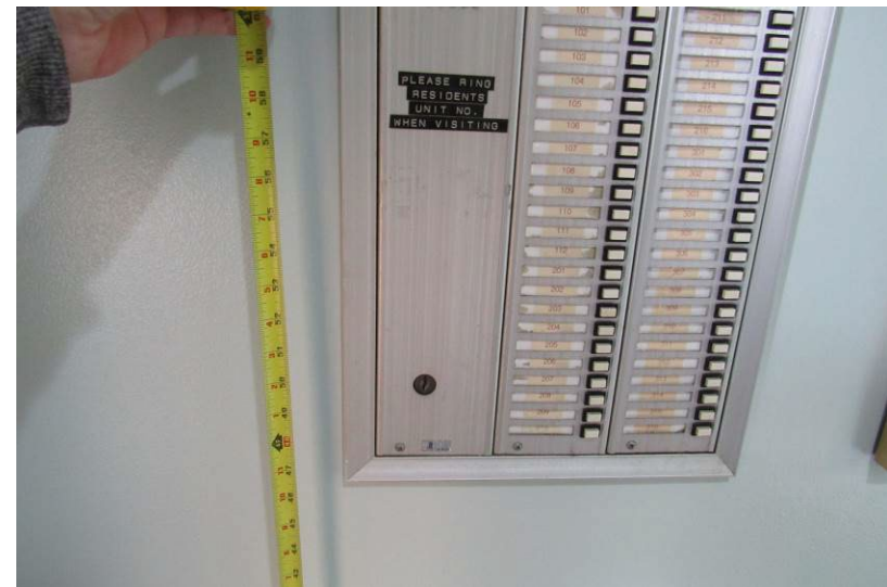
View of entry intercom system regulating visitor entry into building – note select push buttons exceed acceptable UFAS reach range limits
