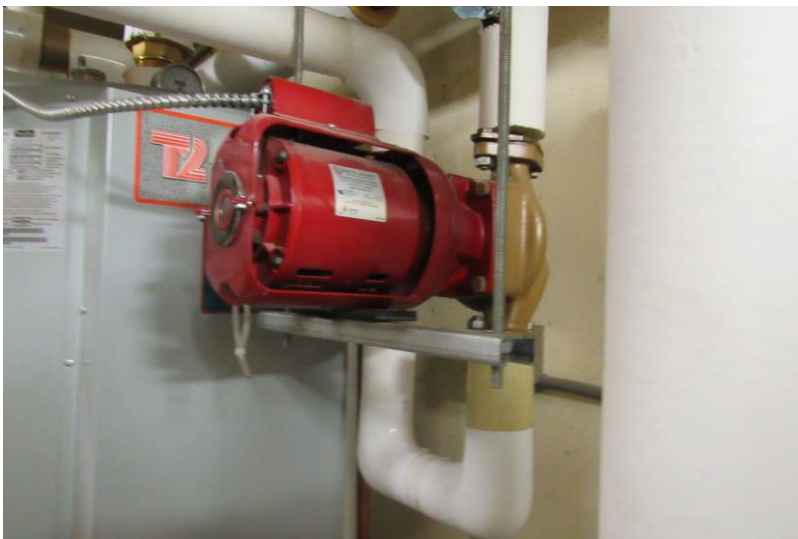
View of fractional horsepower domestic hot water circulation pump
