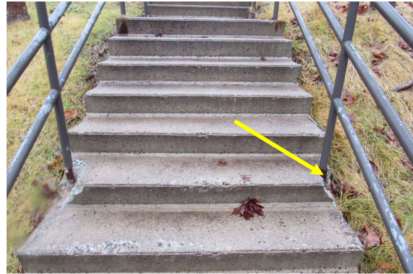
View of concrete steps and railings providing access to bus shelter – concrete spalls and corrosion of metal railing connections observed
