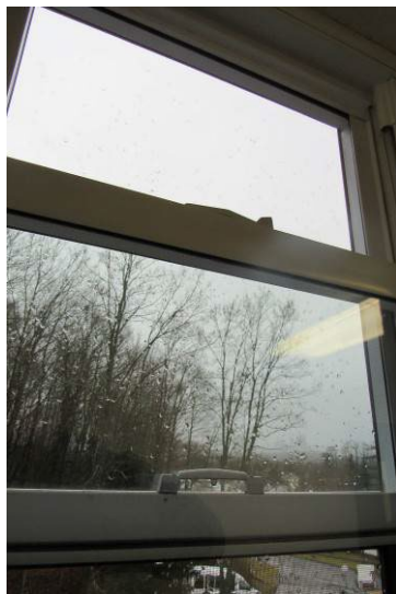
Exterior windows are vinyl-framed double-hung models containing insulating glass units (IGU's) – no widespread failed or cracked IGU's noted during the assessment; isolated windows replaced in past due to water infiltration issues
