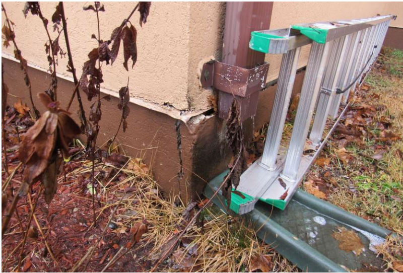
View of apparent displaced section of concrete foundation wall cementitious parge coat as seen at front of building
