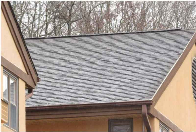
View of architectural asphalt roof shingle conditions as seen from available vantage points – active roof leakage reported at east end of building
