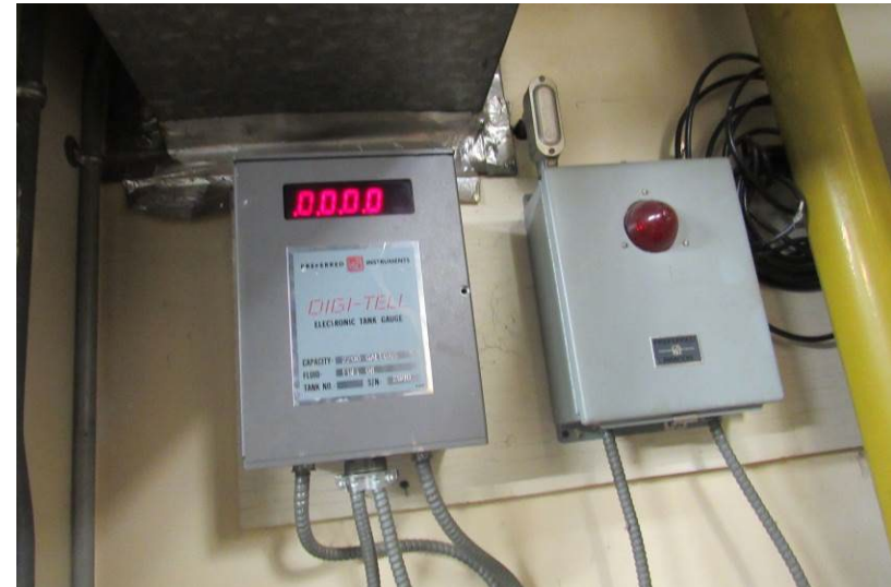
Emergency generator fuel gauge monitor reportedly problematic/not functioning
