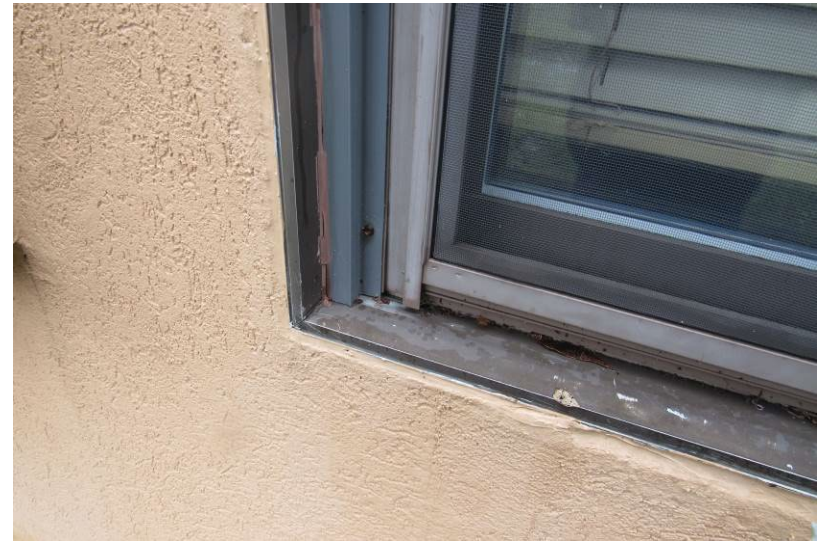
View of deteriorated exterior caulking at window perimeter (cohesive/adhesive failures)
