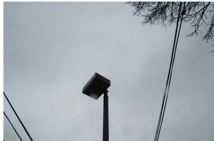
View of typical pole-mounted high intensity discharge (HID) light fixture facilitating site illumination – several light poles exhibit corrosion/weathering
