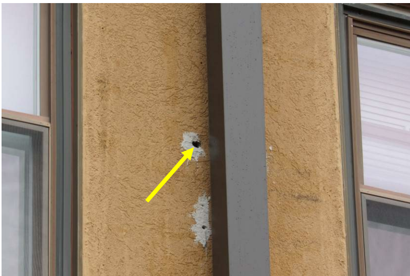
View of voids within exterior insulation and finish system (EIFS) as seen at front elevation – these areas are susceptible to moisture infiltration and subsequent damage to underlying building components/materials
