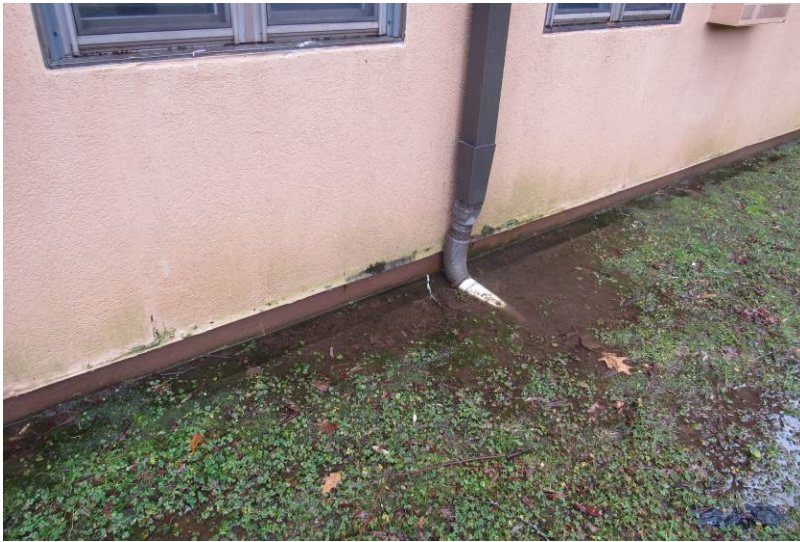
View of rear of building – reportedly poor drainage occurs along portions of this perimeter and may be conducive to water infiltration issues reportedly occurring at ground floor level
