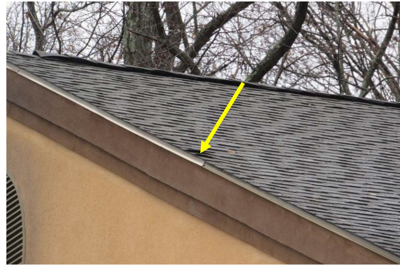
Isolated curled/uplifted shingles noted from available vantage points
