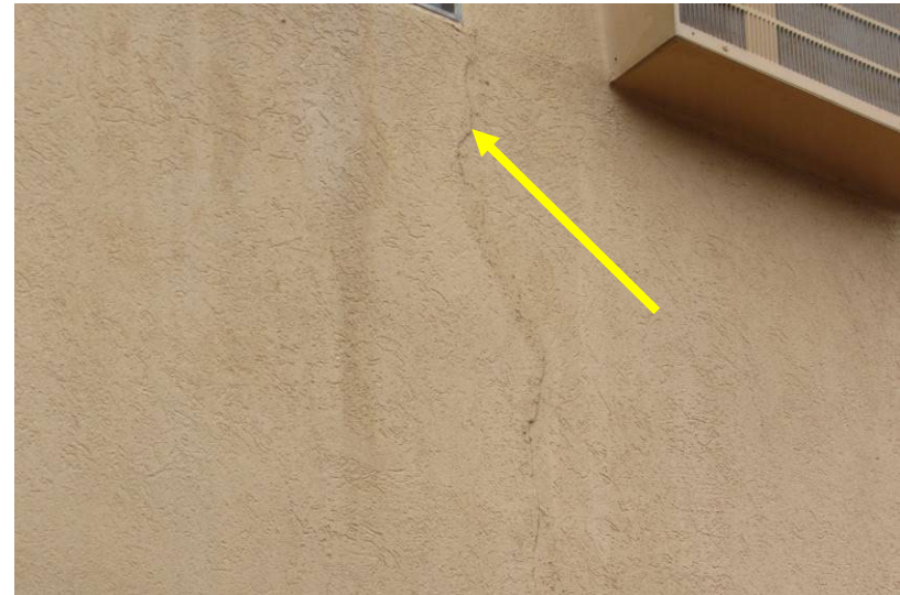
Several areas of cracking observed within EIFS cladding
