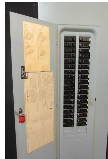
View of typical General Electric circuit breaker panel serving bank of 4 apartment units
