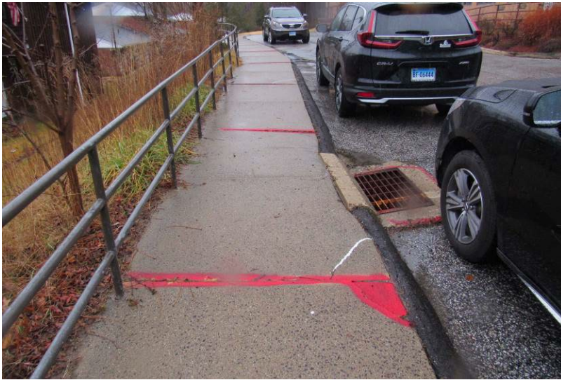
Several areas of unevenness and potential trip hazards observed within concrete flatwork
