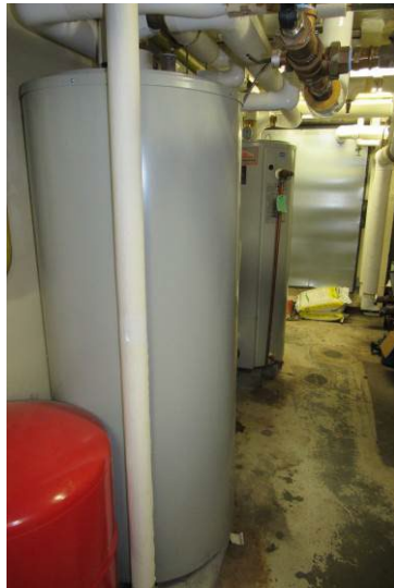
View of indirect-fired domestic hot water (DHW) storage tanks – 119-gallon storage capacity each
