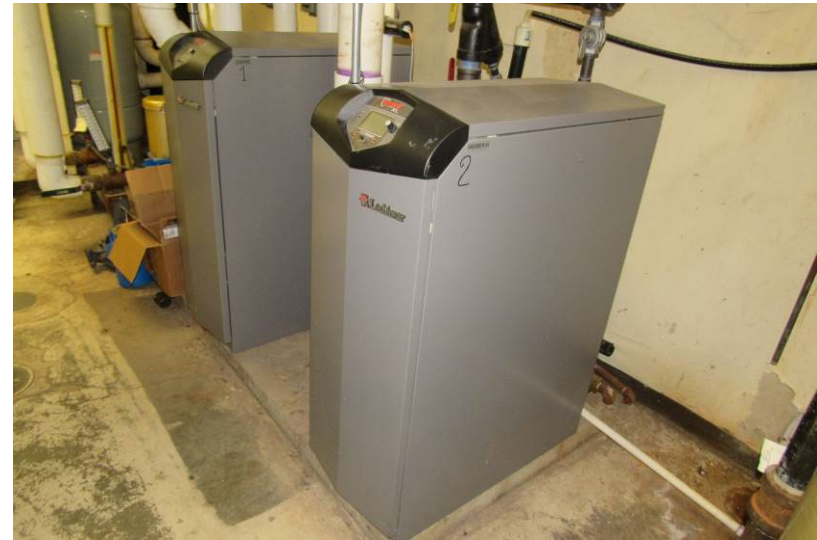
View of Lochinvar natural gas-fired condensing boilers facilitating hydronic heat generation for building – 500 MBH energy input each
