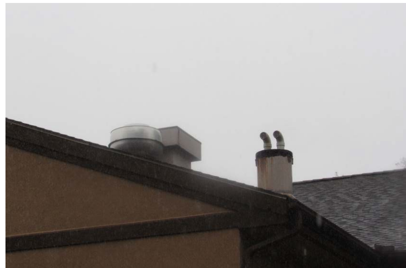
View of boiler flue exhaust; note flues appear to be in close proximity to commercial kitchen ventilation equipment; this condition should be further reviewed and addressed as may be required (i.e., ensure flues are appropriately distanced from kitchen air intake system)
