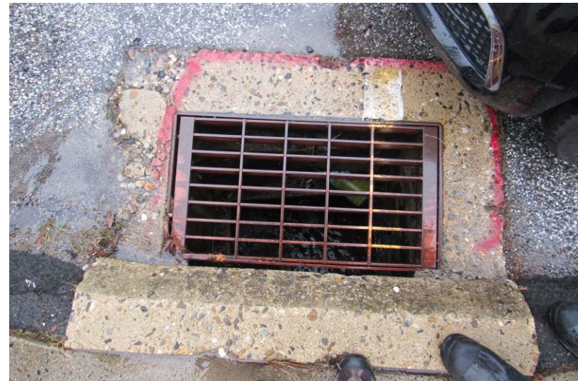
View of catch basin concrete collar exhibiting spalls/deterioration
