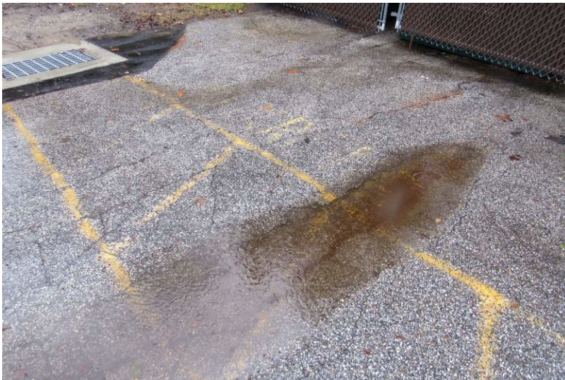
View of pronounced cracking/rutting within asphalt pavement as seen at dumpster enclosure approach – consideration should be given to installing concrete pavement to better withstand loads from waste removal trucks
